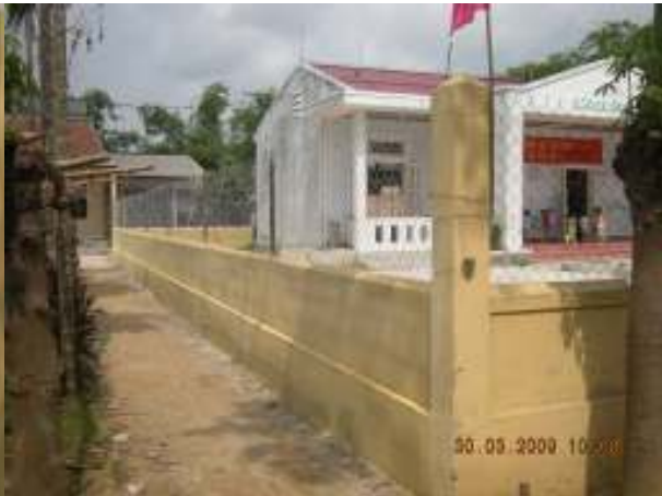
after building fence
