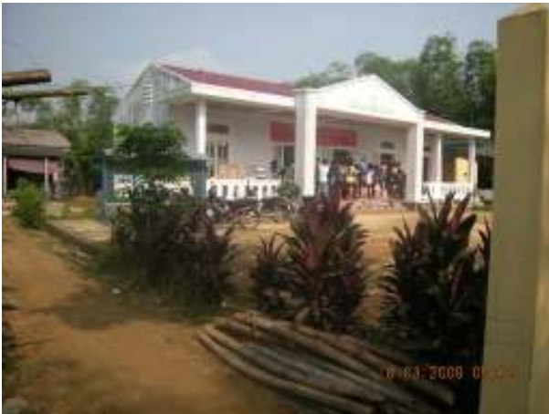
Above: The Kindergarten before
