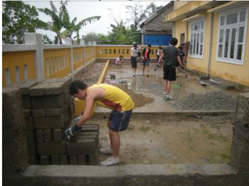
Above: Loading cement blocks to build a kitchen at Loi Nong
