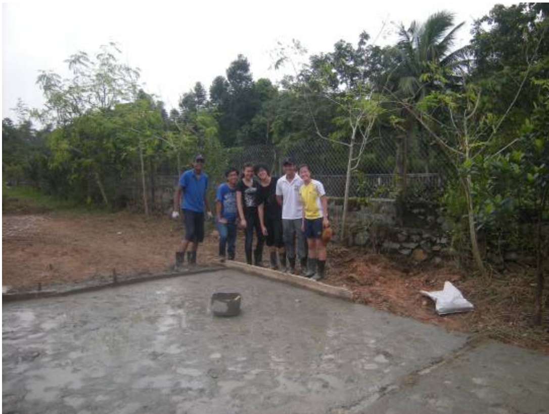
Above: Concreting the courtyard
